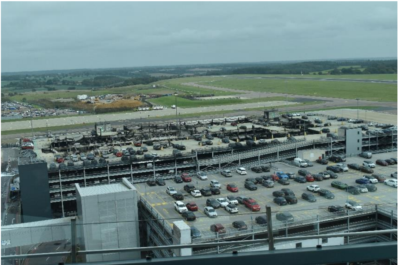
Figure 8 Car Parks 1 and 2 following the fire. Image courtesy of Bedfordshire Police
